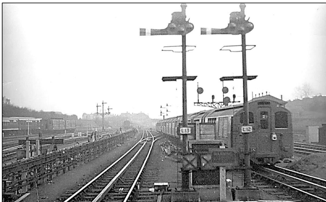
Figure 4: A 6-car train of LER stock leaves Ealing Broadway Central London station. The platform for the Central London was between the District station on the one side and the Great Western on the other side just as it is today. This is the only photo I recall showing LER stock running on the Central London 3-rail system. The photo dates from between November 1938 and May 1940 when the 4-rail installation was completed. Note the GW
